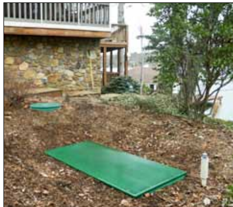
A typical AX20-RT system installation. Note the system's small footprint. The AX20-RT measures 8.5 x 6 x 5.2 ft (2590 x 1830 x 1575 mm).
